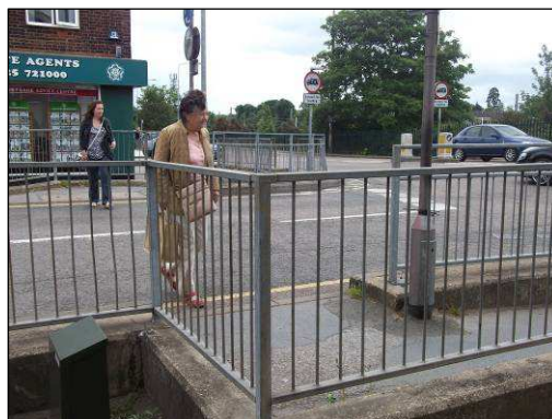
Pedestrian guard railing in Flitwick
